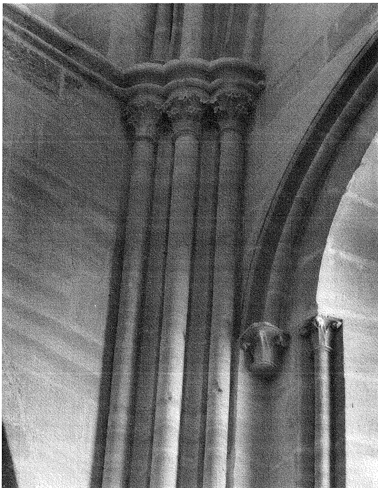
Figure 44. Cuenca cathedral, interior of south transept facade, southeast corner (Photo: author)
