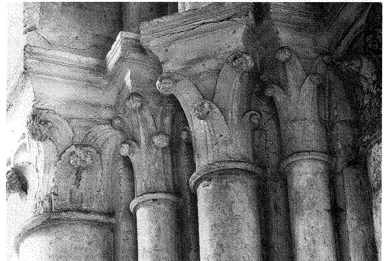
Figure 35. Noyon cathedral, entry arch to north transept from north aisle of nave, south side, pier capitals (Photo: author)
