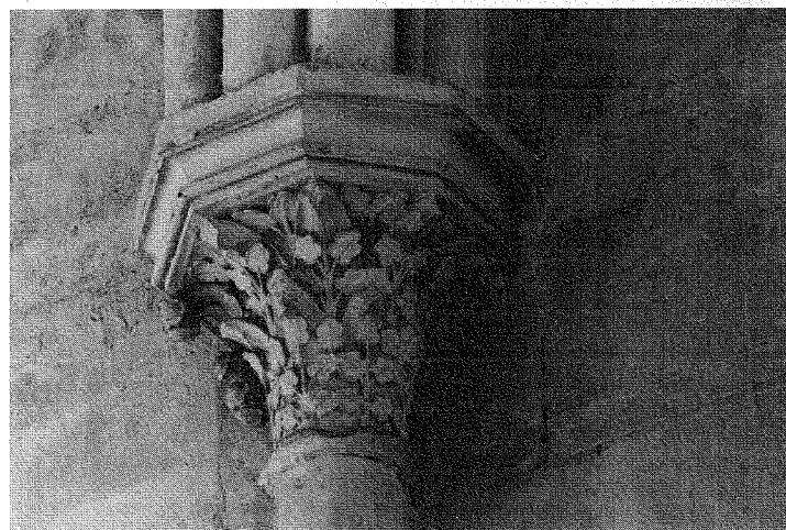
Figure 31. Las Huelgas, Santa María la Real, outer chapel of north transept, capital of corbeled respond on south wall (Photo: author; copyright: Patrimonio Nacional)
