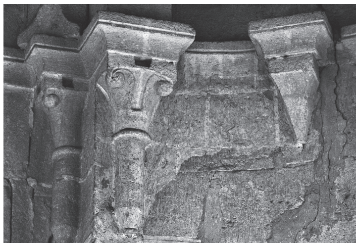
Fig. 17. Santa María de Carrizo, north apse, corbeled supports on north side of vault, c. 1210. (photo: author)
